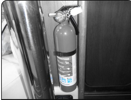
Photo 8: ABC Fire Extinguisher
