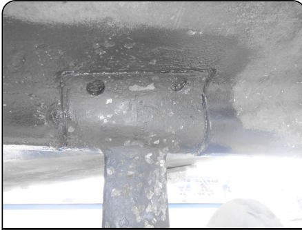
Photo 130: Paint peeling in areas and was recoated with ablative bottom paint.
