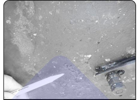
Photo 132: Paint peeling in areas and was recoated with ablative bottom paint.
