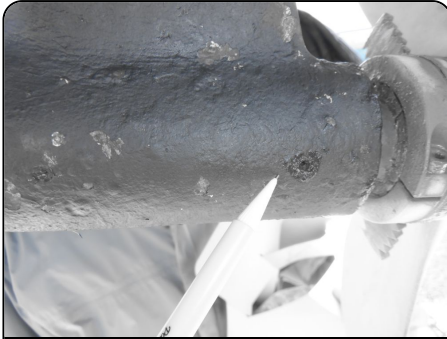
Photo 123: Cutless Bearing set screws in place
