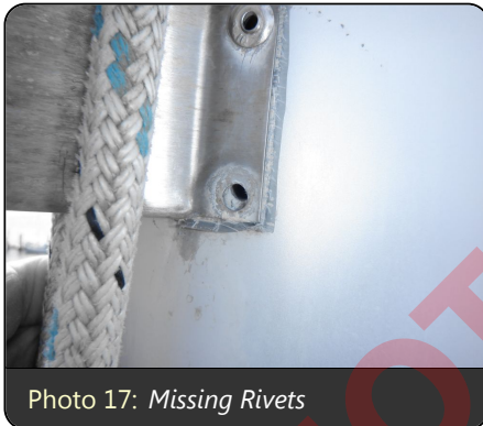
Photo 18: Missing Rivets
